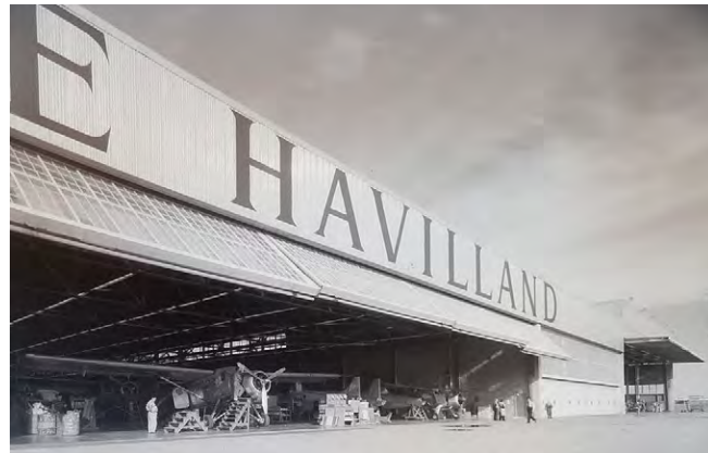
Figure 2: c. 1958 photo of Bays 2, 3 and 4
