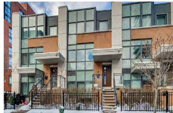
Figure 61: 16 Cole Street Townhomes, Toronto
