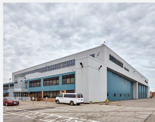
Figure 82: Existing Bay 12 building
