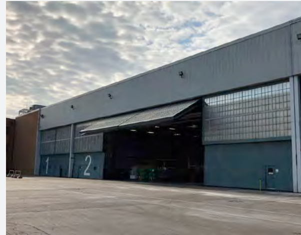
Figure 80: Existing hangar bays 1-3
