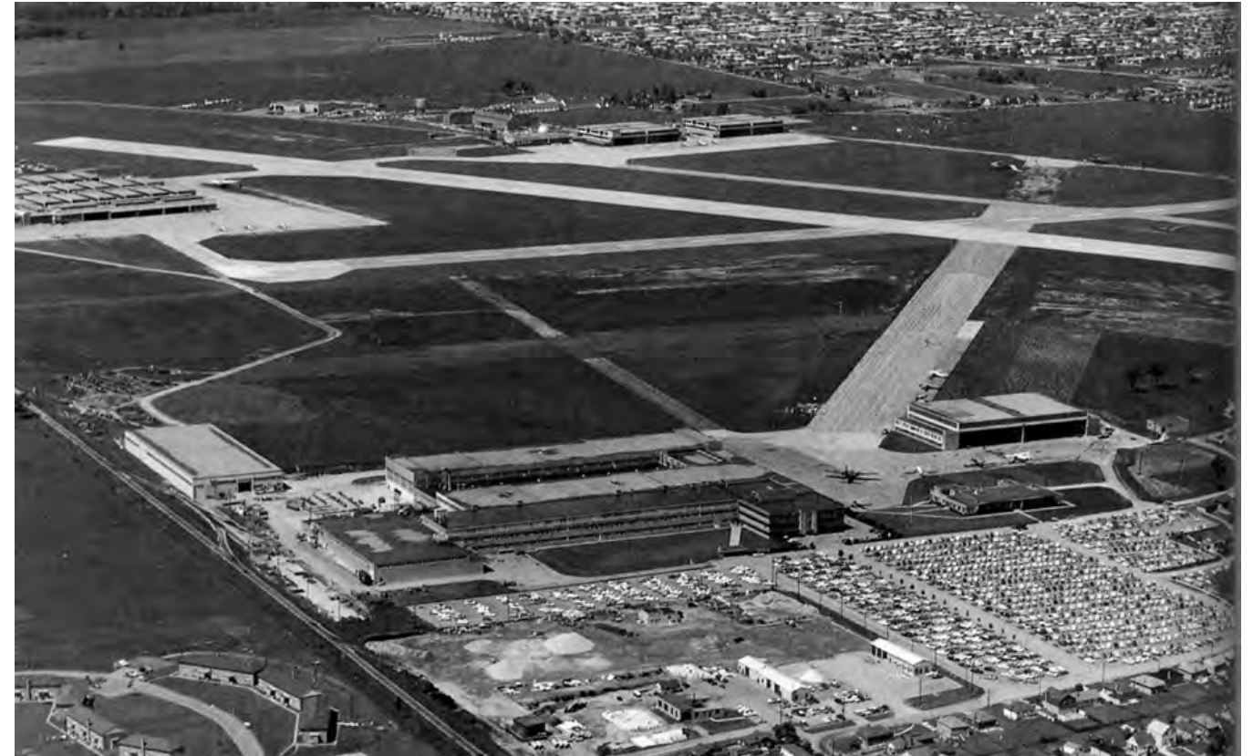
Figure 3: Late 1950s or early 1960s aerial image of the Taxiway West District lands
