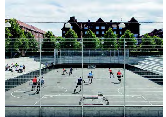
Figure 93: Floodable multi-use court in Enghave Climate Park, Copenhagen
